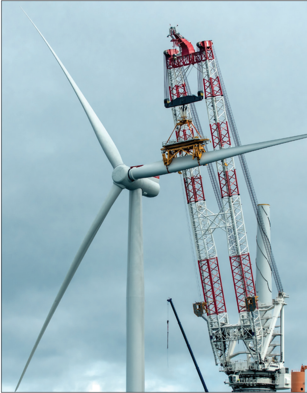
Above: Specialized workers use cranes to erect offshore wind turbines. Legislation passed this year will advance training for offshore wind workers in Virginia. Shutterstock.
