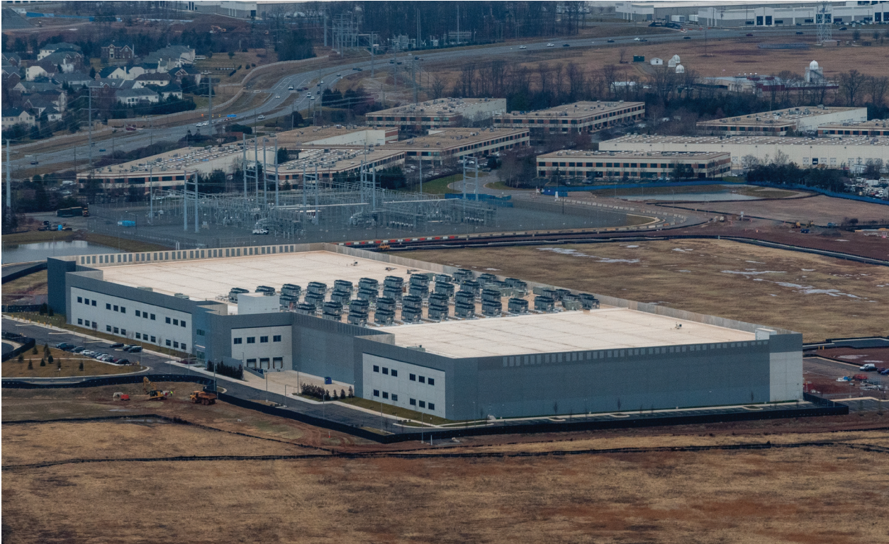
Aerial view of a hyperscale data center in the Dulles Technology Corridor in Loudoun County, which houses the highest concentration of these facilities in the world. Shutterstock.
